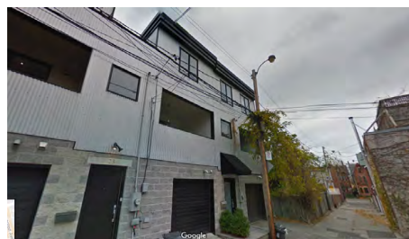
23 Skey Lane. Photo credit: Google Maps
